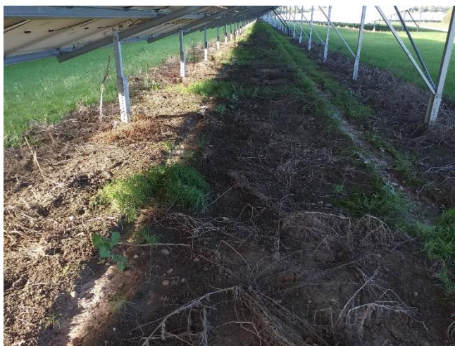
Figure 6: Channels created by panel runoff within 12 months of site operation commencing
